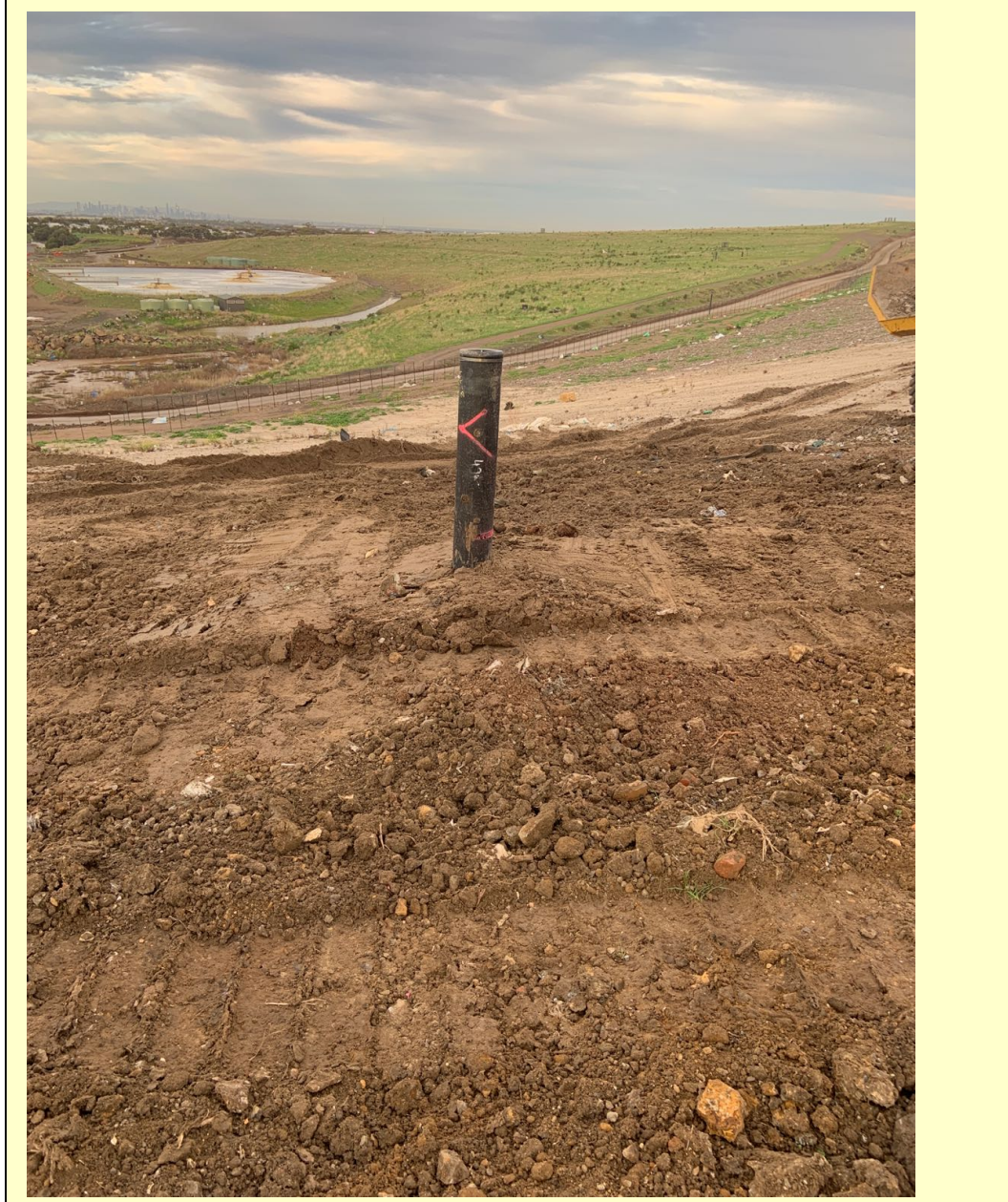
Photo - Take Photo of Completed Well
